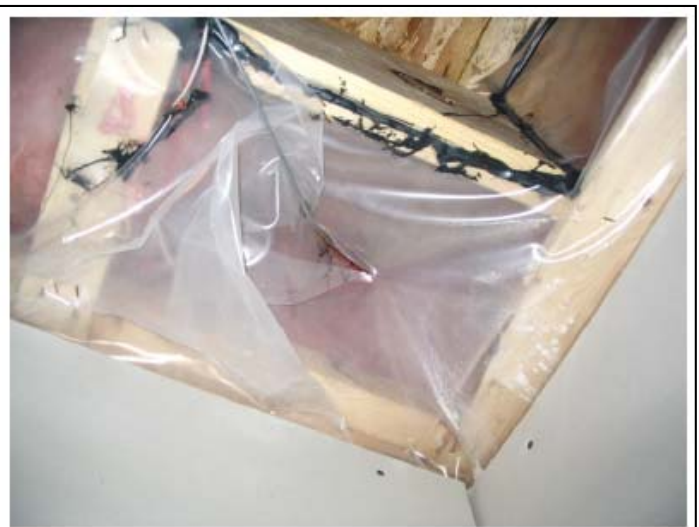
Install security wiring before insulating.
