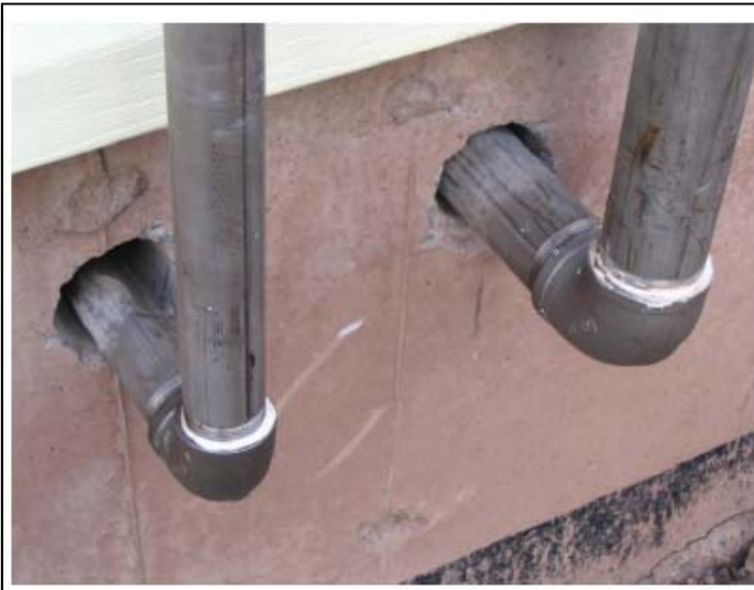
Oil filler pipes should be sealed from the outside and foamed from the inside.
